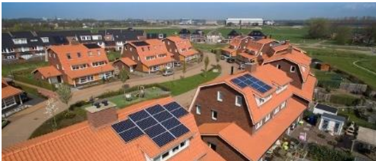
Hoog Dalern, all-electric district, Gorinchem
